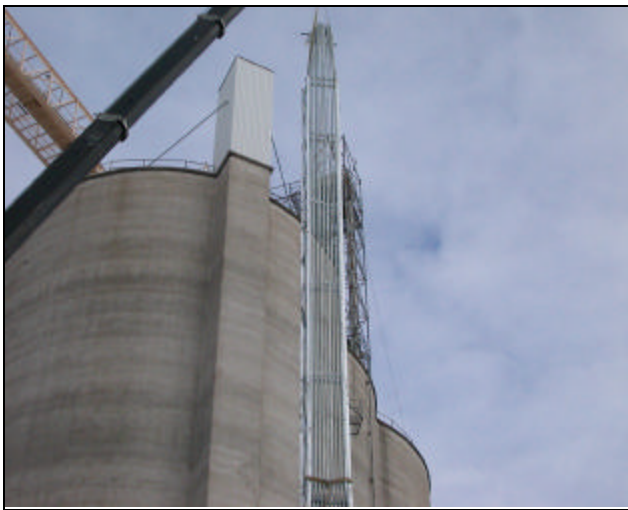
Hoisting of conduit rack onto silo
