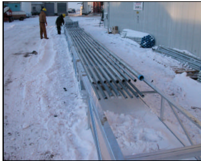
Ground level assembly of a 135 foot conduit rack
