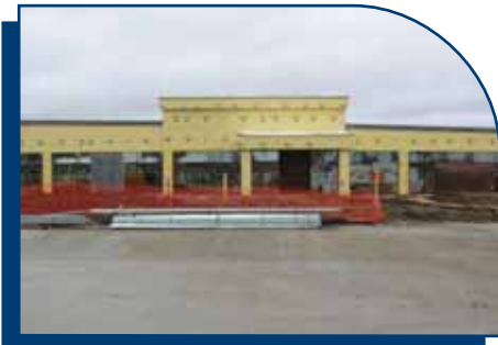
Progress Continues on the East Campus Expansion
