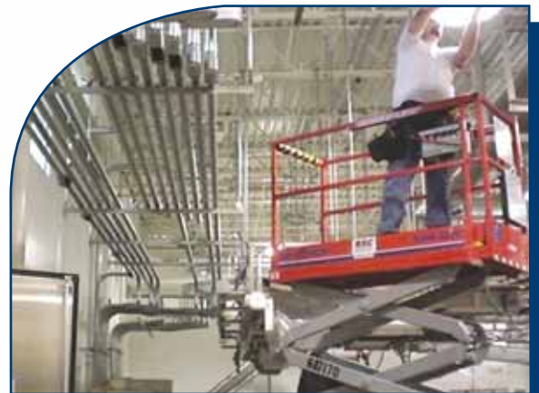
Initial Conduits over Packaging Area Panels
