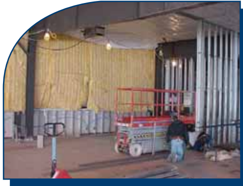
Workers Install Steel Studs for the East Campus' Interior Walls
